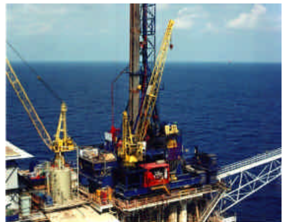
Rigged-up on platform without docking in international port.
